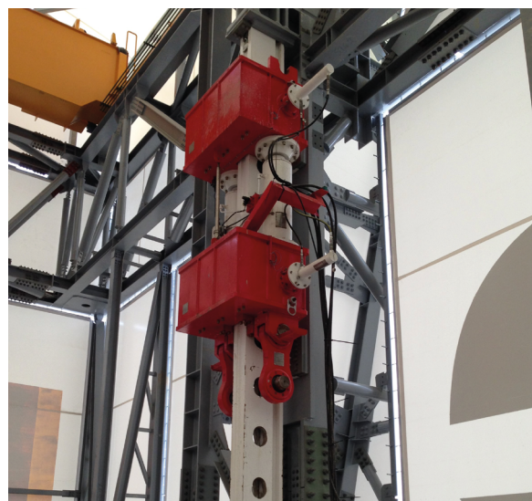
→ FIGURE 8: Dorman Long jacking system
