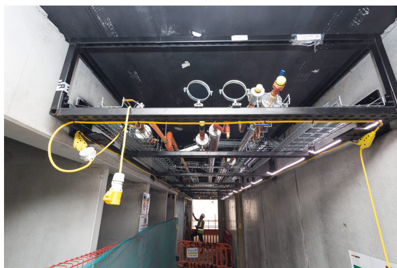
↖ FIGURE 10: Twin-wall core with modular MEP 'H-frame'
